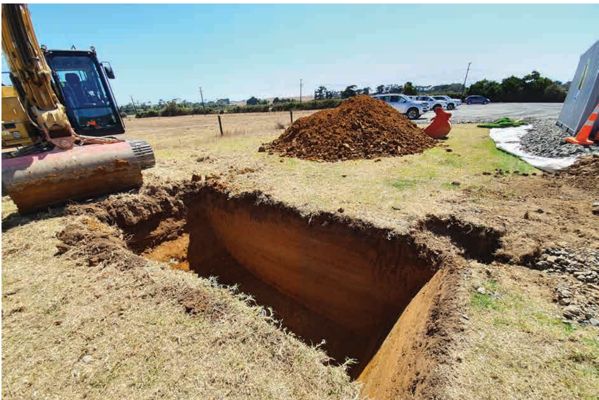
Figure 6. View east of septic tank cut behind farmhouse.
